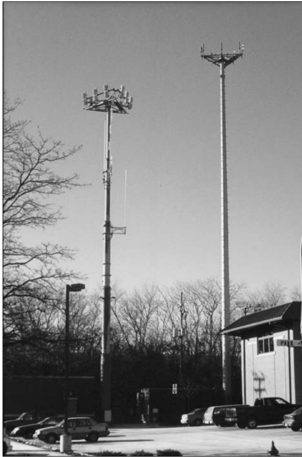
Figure 3-17 A cellular telephone tower
