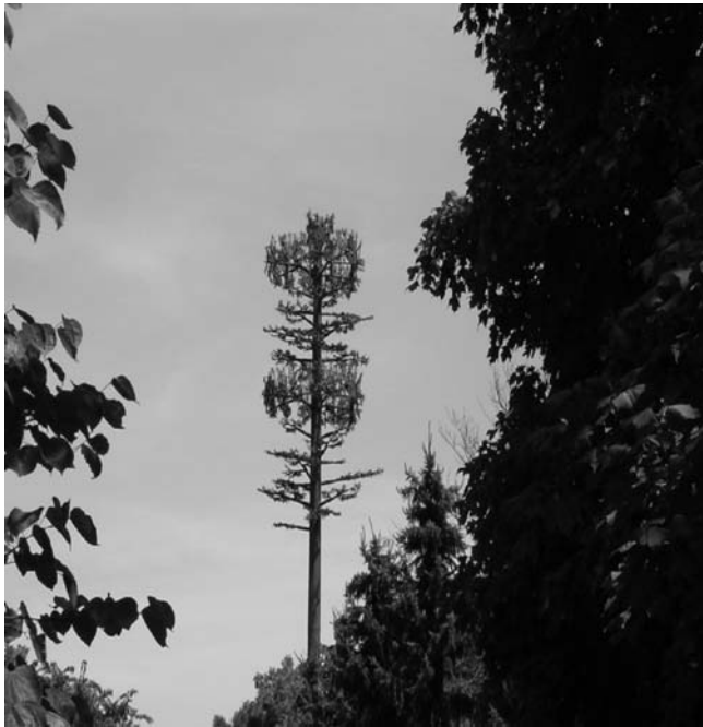
Figure 3-18 Cell phone towers disguised as trees
