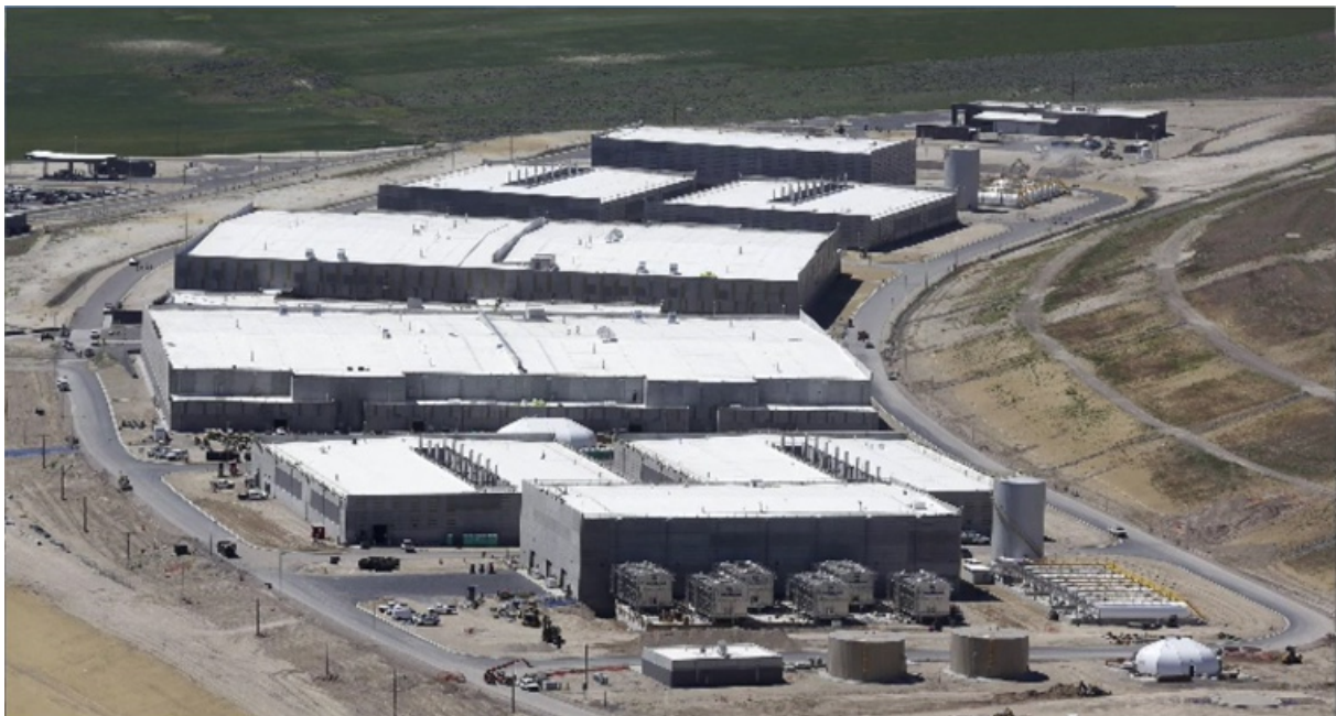
Data center in Utah
