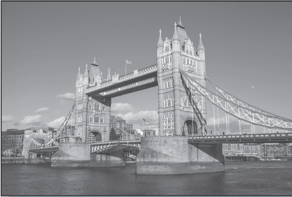
Figure 10.1 London Tower Bridge.
