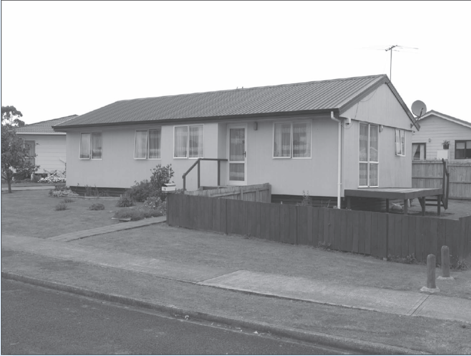
Figure 8.1 The house built in less than 4 hours.
