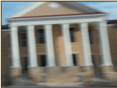
Due to a rolling shutter distortion, the pillars of the building appear to be leaning.
