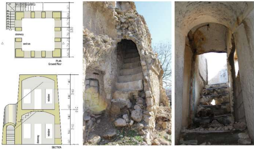
Fig. 5. Doors and windows transformed to wall niches used as shelves, cupboards or fire places.
