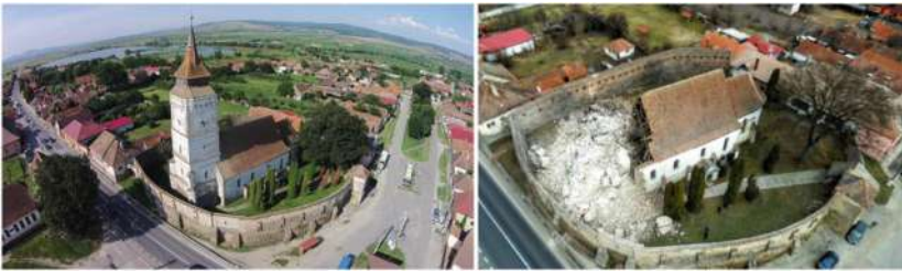
Fig. 3. Rotbav Fortified Church before and after collapsing in 2016.
